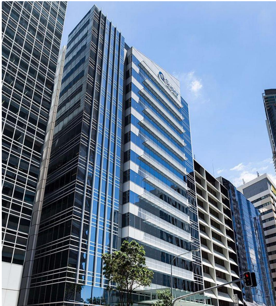
Figure 112 - 70 Eagle Street, Brisbane, Australia
